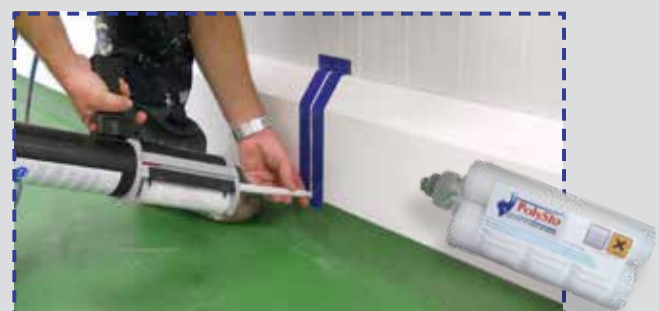
PolySto OP30RB SaniCoat with epoxy floor coving applied into a rebate and finished with PolySto HygiSeal.
