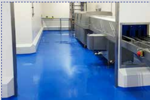
PolySto IP40RB Natural with epoxy floor covering applied into a rebate.
