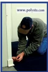
Apply a 'PolySto Hard Fix Glue' line on the floor and to the back of the corner.  $\label{eq:constraint} % \begin{subarray}{ll} \end{subarray} %$
