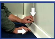
Push the kerb up against the wall and level immediately (with pinch bar and suction cups).
