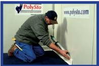
A drying period of at least 24 hour is required for the adhesive.
