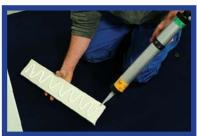
After installing the end pieces and angles, install the straight lengths of kerbs in between in the same way.
